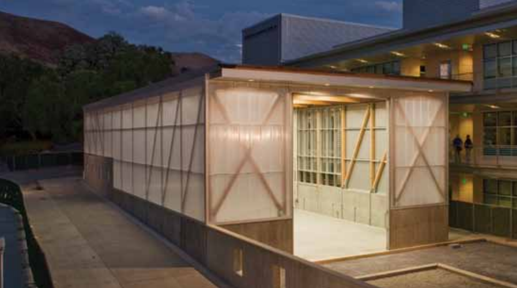
SST with Heavy Timber Braced Frames at Dusk.
