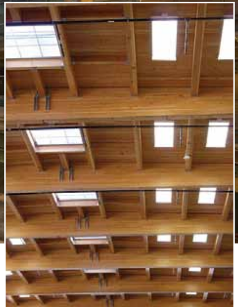
Interior View of Heavy Timber Roof.
