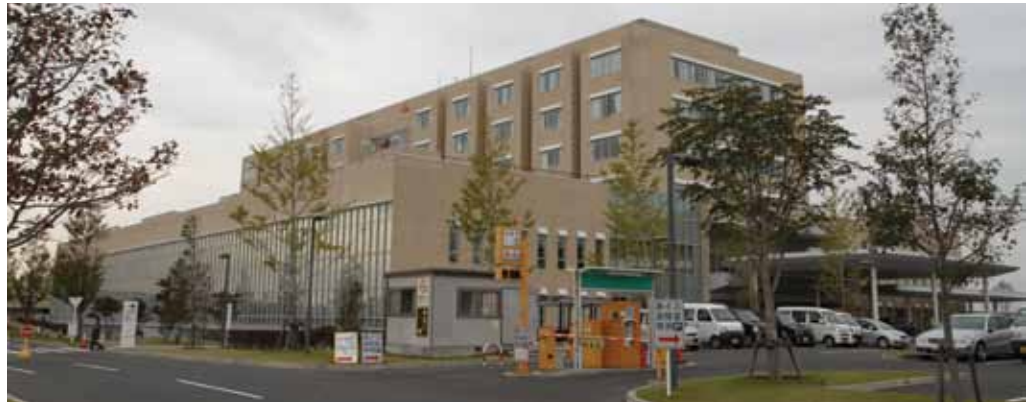
The seismically-isolated Ishinomaki Red Cross Hospital, about 75 miles (120 km) from the epicenter of the M9.0 Great Tohoku Earthquake of March 11, 2011, was undamaged, and fully-operational throughout and after the earthquake and subsequent tsunami. Courtesy of SIE, Inc.
