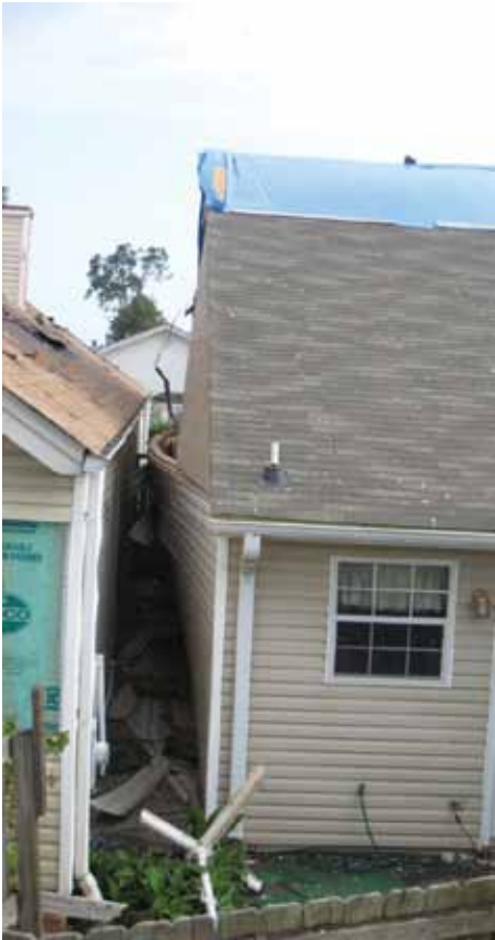
Figure 4: Pressurized exterior wall.
