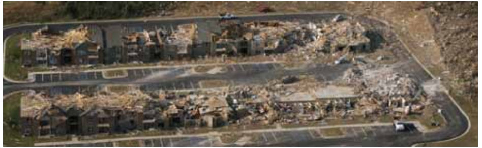
Figure 5: Catastrophic damage at apartment complex.
