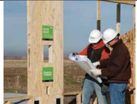
Wood pre-fabricated shear panels can accommodate high lateral loads in narrow wall segments.
