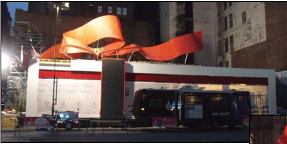
Above: Bank of America Gift Box, a temporary 350 square foot pavilion on Fifth Ave. in New York City, built as a “gift” to the people of New York for the 2007 holiday season. McLaren engineered the temporary building structure, temporary foundation and rooftop ribbon assembly. Courtesy of McLaren Engineering Group.
