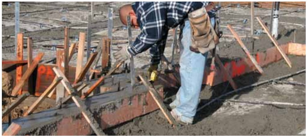
Figure 3: Adjusting a Strap in the Footing Prior to Pouring the Slab.
