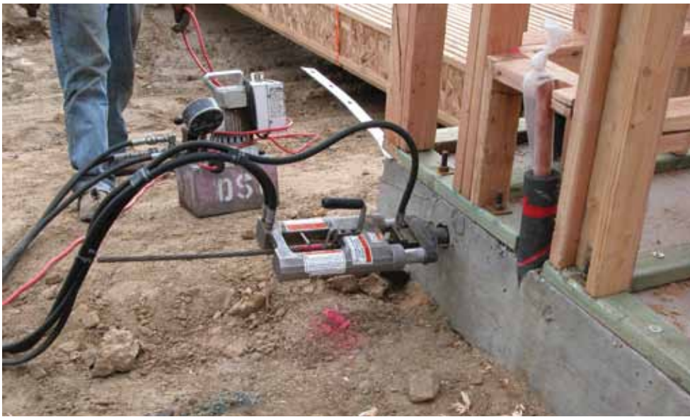
Figure 4: Typical Stressing Equipment.
