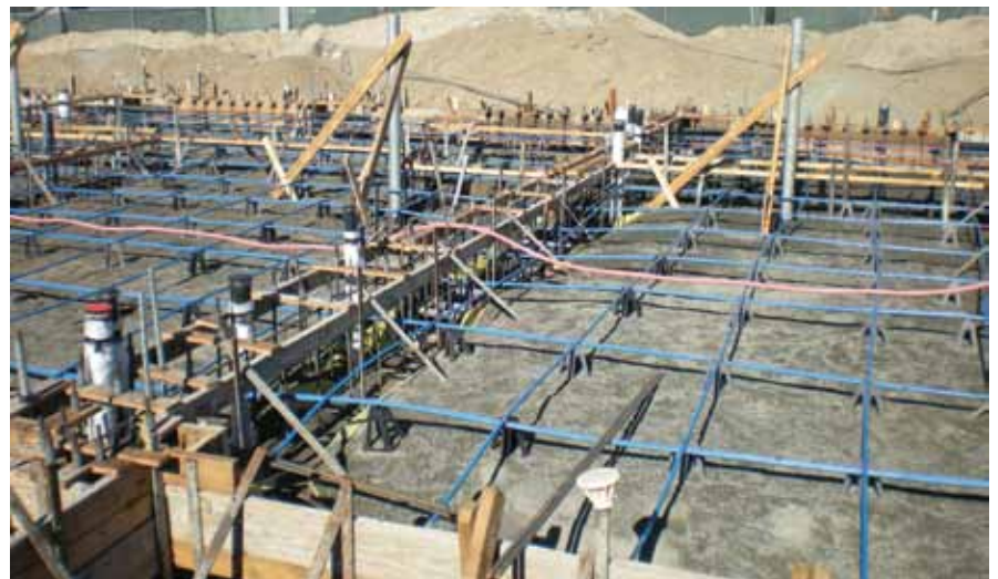
Figure 2: Plastic Chairs Used to Support the Tendons.
