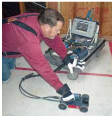
Figure 2: Scanning Slab to Locate Existing Strands.
