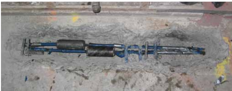
Figure 4: Coupler Used to Re-Connect Broken Strands.
