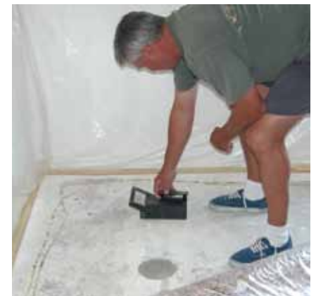
Figure 3: Pacometer (Metal Detector) used to Locate Existing Strands.
