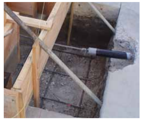
Figure 5: New Pad Footing in an Existing Post-Tensioned Foundation.
