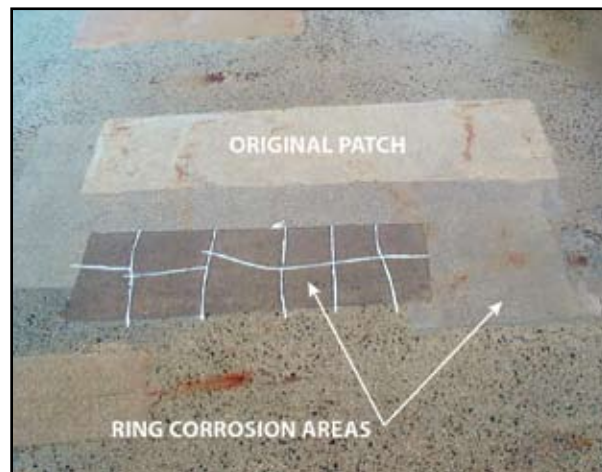
Figure 3: Ring corrosion.
