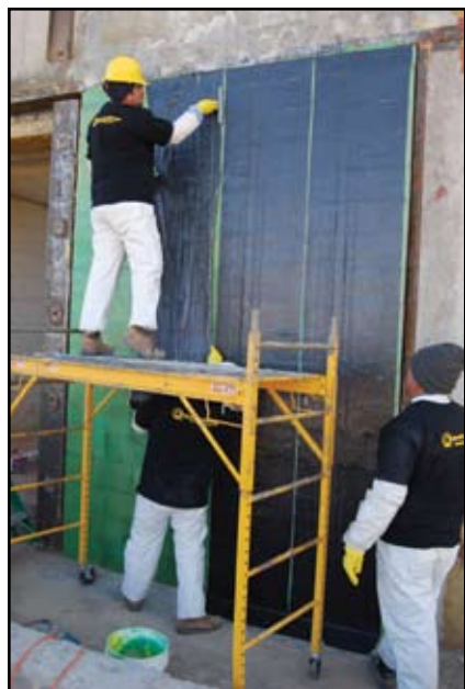
Figure 1: CFRP fabric installation on URM wall.
