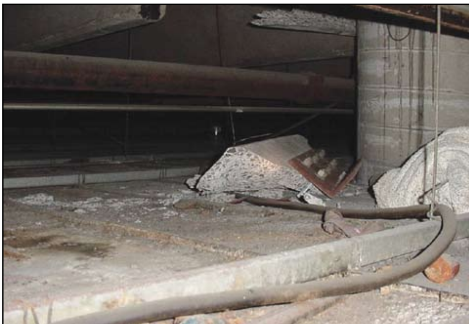
Figure 4: Failed and fallen steel angle bracket connection bolted to concrete.
