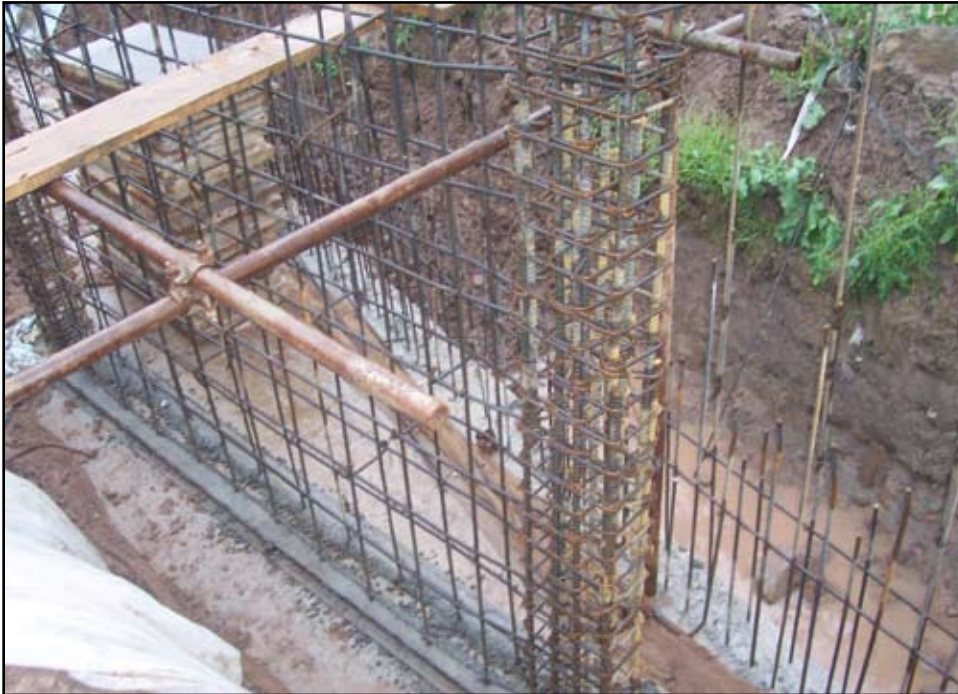
Figure 4b: Construction Photo of a Shearwall Rebar Cage.
