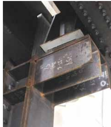
Figure 2: Slide-Bearing Connection for Seismic Movement Joint.
