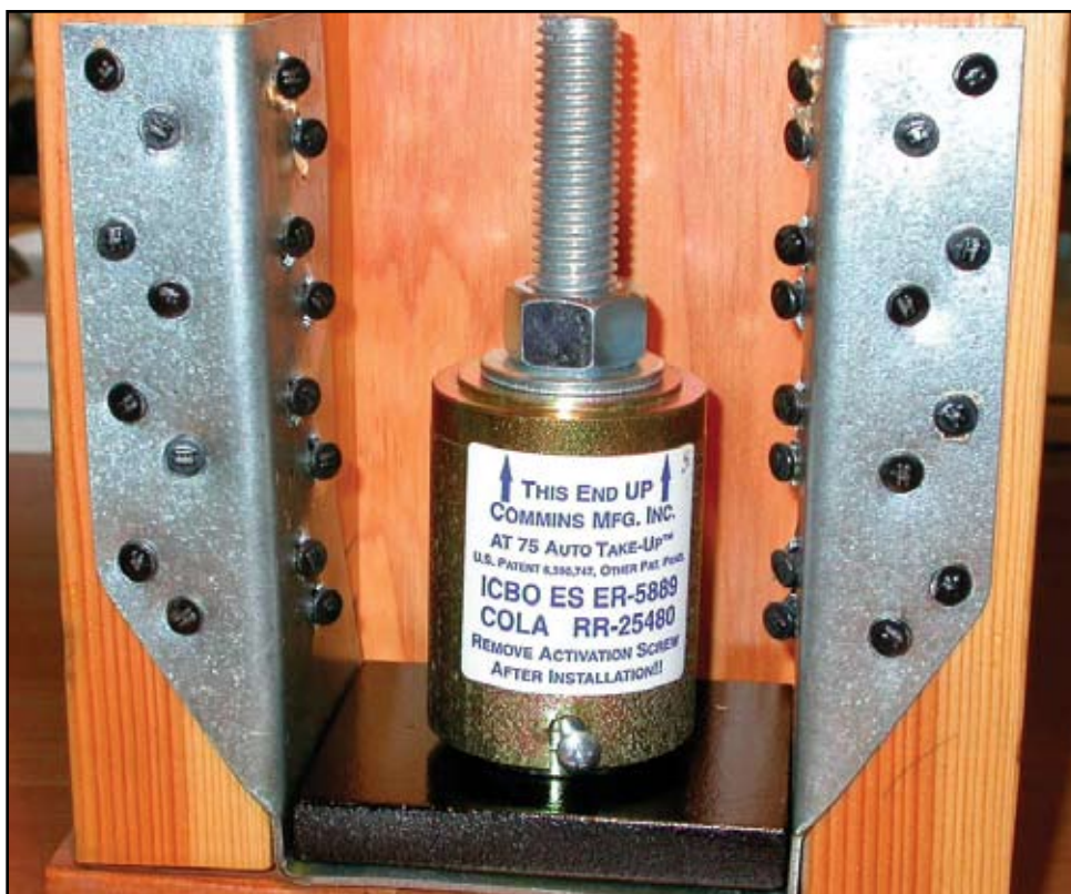
Figure 6: A nailed-on concentric hold down.
