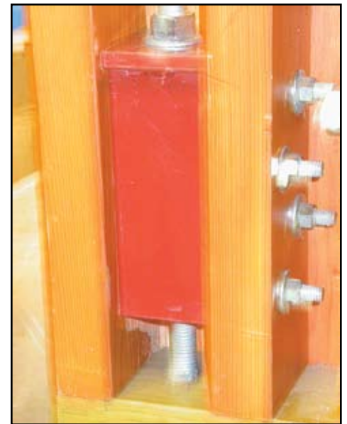
Figure 5: A bolted concentric hold down.
