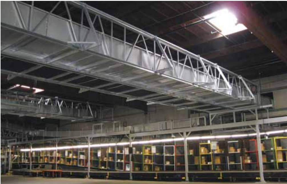
Figure 1: TrusSteel CFS Truss Bridge over drive-thru bay.
