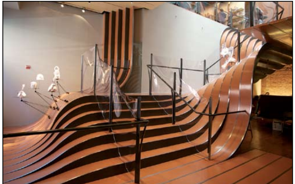
Figure 6: Lighting and product displays are connected to the 1.25" plates using high-strength magnets.
