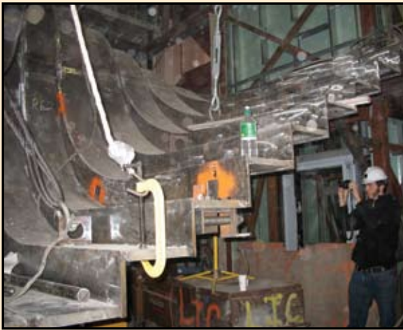
Construction: Upper mezzanine and cantilever, suspended over the construction photographer.
