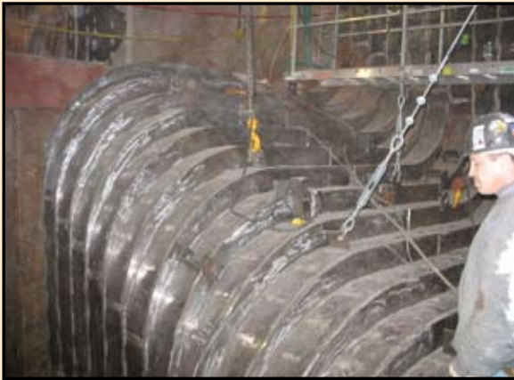
Construction: Erecting the top flight at second floor.
