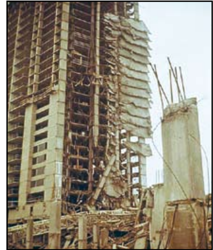
Figure 1: The progressive collapse of the middle portion on this building in Baileys Crossroads, caused by premature formwork removal, resulted in 14 fatalities. Courtesy of the National Institute of Standards and Technology.
