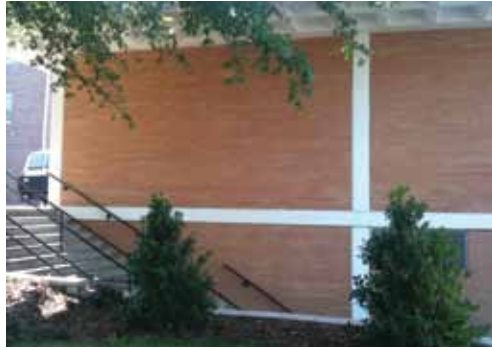
Figure 1: Clay masonry infill with concrete frame.
