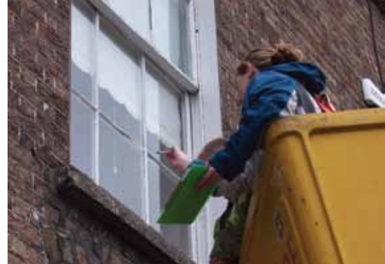
Figure 1: Inspection of Masonry Façade. Courtesy of Dr. Debra F. Laefer.
