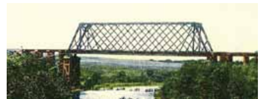
Figure 14: A Hilton, riveted, wrought-iron lattice truss over the James River near Redfield, South Dakota. Note the vertical truss member at the hip joint. Author's post card collection.
