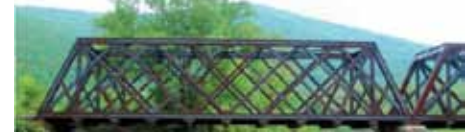
Figure 20: Norfolk and Southern Railroad Hilton Lattice Truss, over Seeley Creek, near Elmira, New York. Courtesy of Nathan Holth at historicbridges.org .
