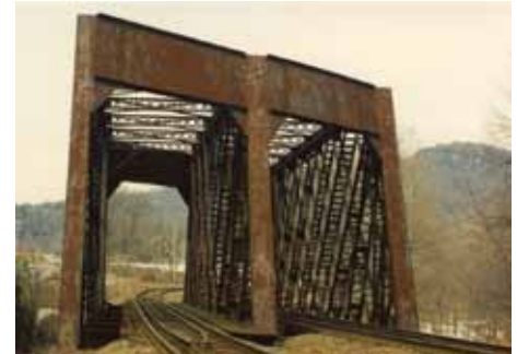
Figure 21: Lattice Railroad Trusses. Hillburn, New York. Courtesy of David Guise.
