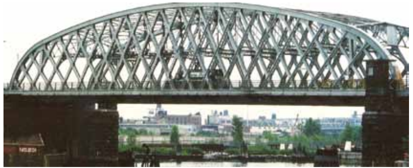
Figure 16: Willis Avenue Bridge. Over the East River. New York City, 1901. Courtesy of David Guise.
