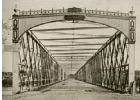
Figure 19: 1877 Lattice truss over the Connecticut River. Springfield Massachusetts. Courtesy of Springfield Museum. Provided by Cliff McCarthy.
