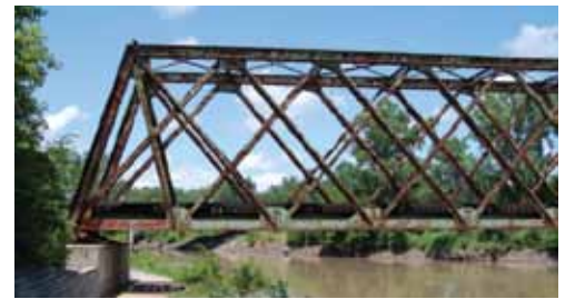
Figure 13 (continued from figures shown in the August article): A Triple Warren Union Pacific Railroad Bridge over the Blue River near Manhattan, Kansas. Courtesy of James Baughn, webmaster at bridgehunter.com .
