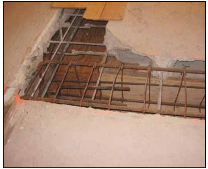
Strengthening of existing slab (Slag Block System).
