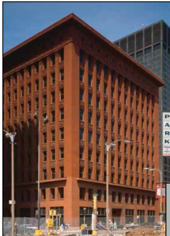
Wainwright Building (St. Louis, Mo.). Example of steel skeleton framing clad with brick masonry.
