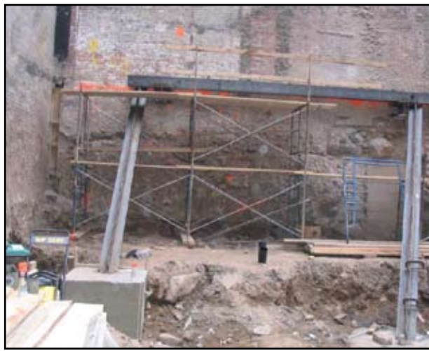
Figure 4: Stabilization of party wall following demolition.
