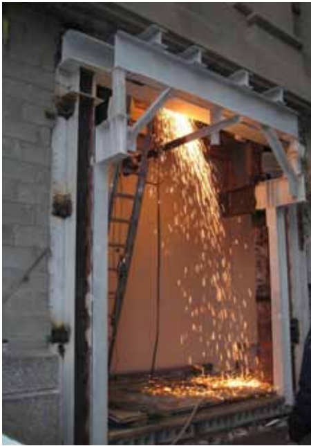
Figure 5: (Construction administration) Changes during construction also require unique solutions. Designers, working closely with the contractor, analyzed new conditions requiring the raising of a storefront elevation, resulting in the existing lintel system, which included a complicated shoring procedure.
