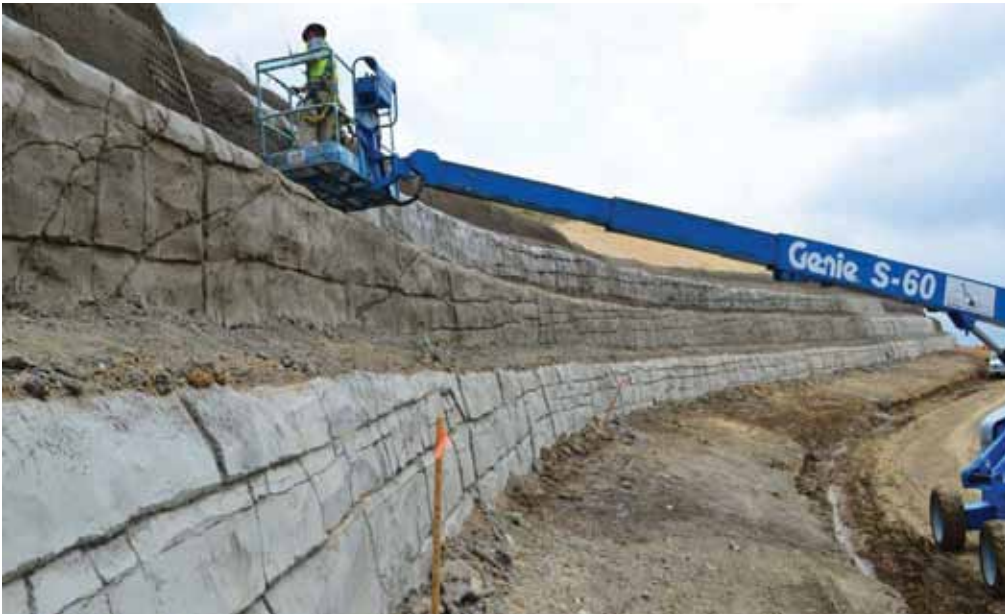
Soil nail wall construction.
