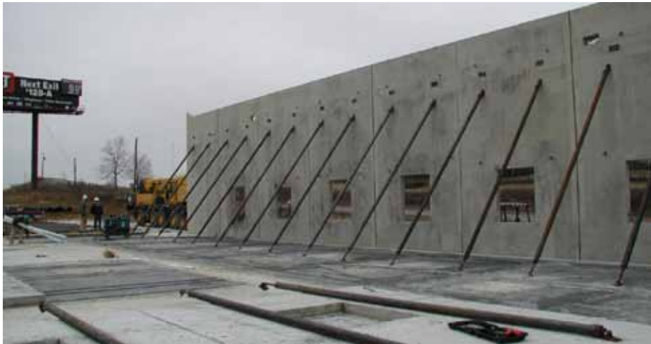
Erected wall panels braced to the slab on grade.
