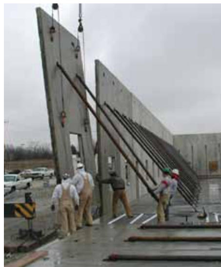
Wall panel erection in progress.
