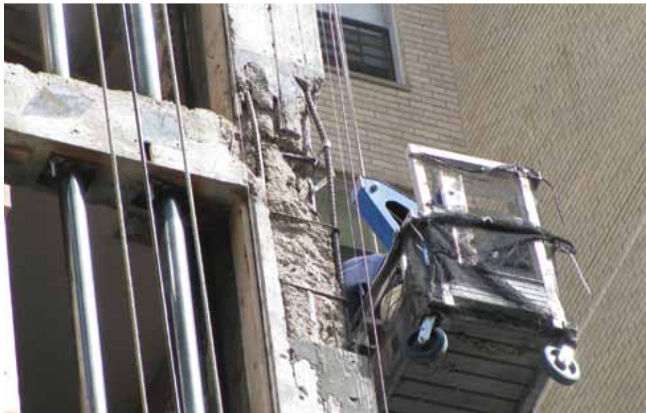
Figure 3. Buckled reinforcing steel bar.
