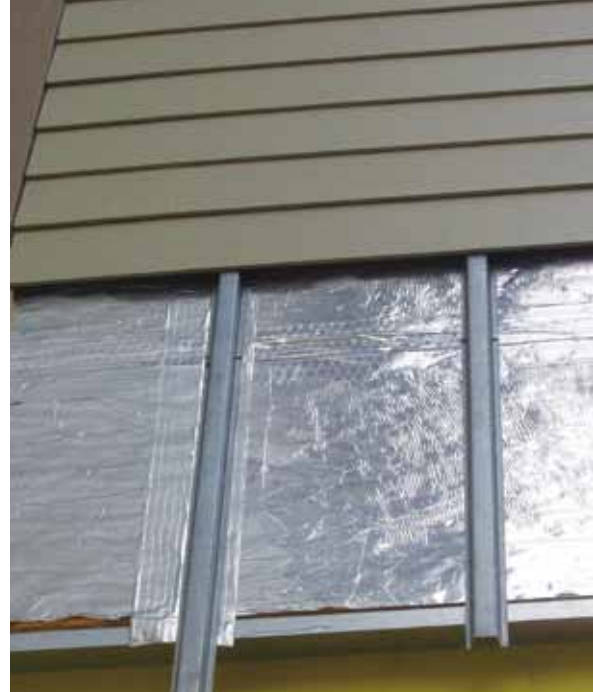
Figure 1: Foam insulation over a building frame using steel hat channels over the foam to attach the cladding.
