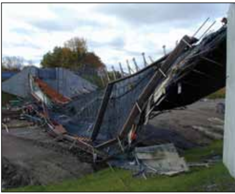
Figure 4: Marcy Pedestrian Bridge in Utica, NY.
