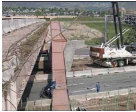
Figure 5: I-70 Overpass at Golden, CO.
