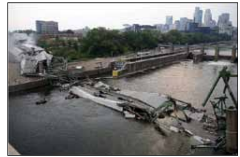
Figure 6: I-35W Bridge over the Mississippi River.
