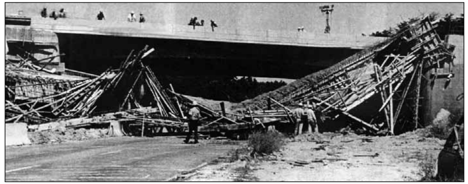
Figure 8: Baltimore-Washington Parkway. Side view of collapse. (From ENR, September 7, 1989)
