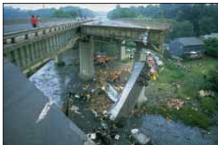
Figure 2: I-95 Bridge over the Mianus River in Connecticut.
