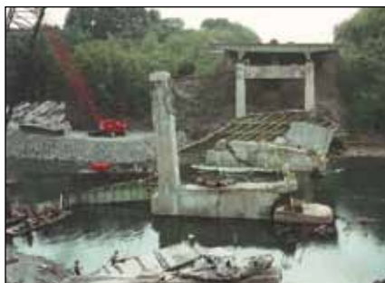
Figure 3: New York State Thruway Bridge over the Schoharie River.
