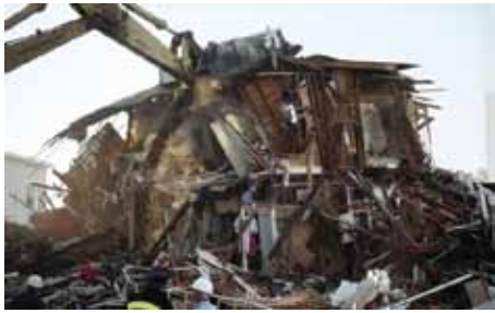
Figure 8: Collapsed wood frame buildings following the Loma Prieta earthquake.
