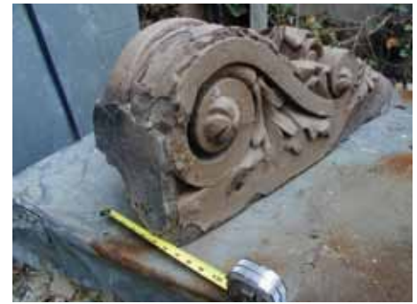
Figure 10: Decorative pediment fallen from a building façade in Brooklyn, NY.
