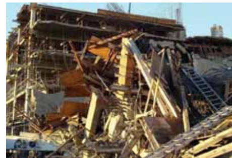
Figure 4: Collapsed Berkman Plaza.
