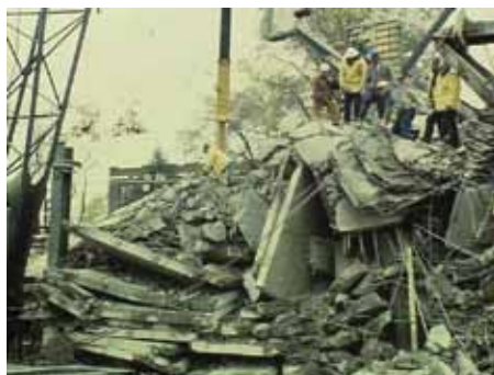
Figure 3: Collapsed lift-slab buildings at L’Ambiance Plaza.
