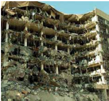
Figure 9: Heavily damaged Murrah Federal Office Building following its bombing.
