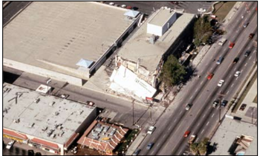
The wide range of damage at the epicenter of the 1994 Northridge earthquake illustrates that not all existing, non-compliant buildings are dangerous. One building partially collapsed while others of similar vintage remained usable. Courtesy of Lloyd Cluff, 1994.
