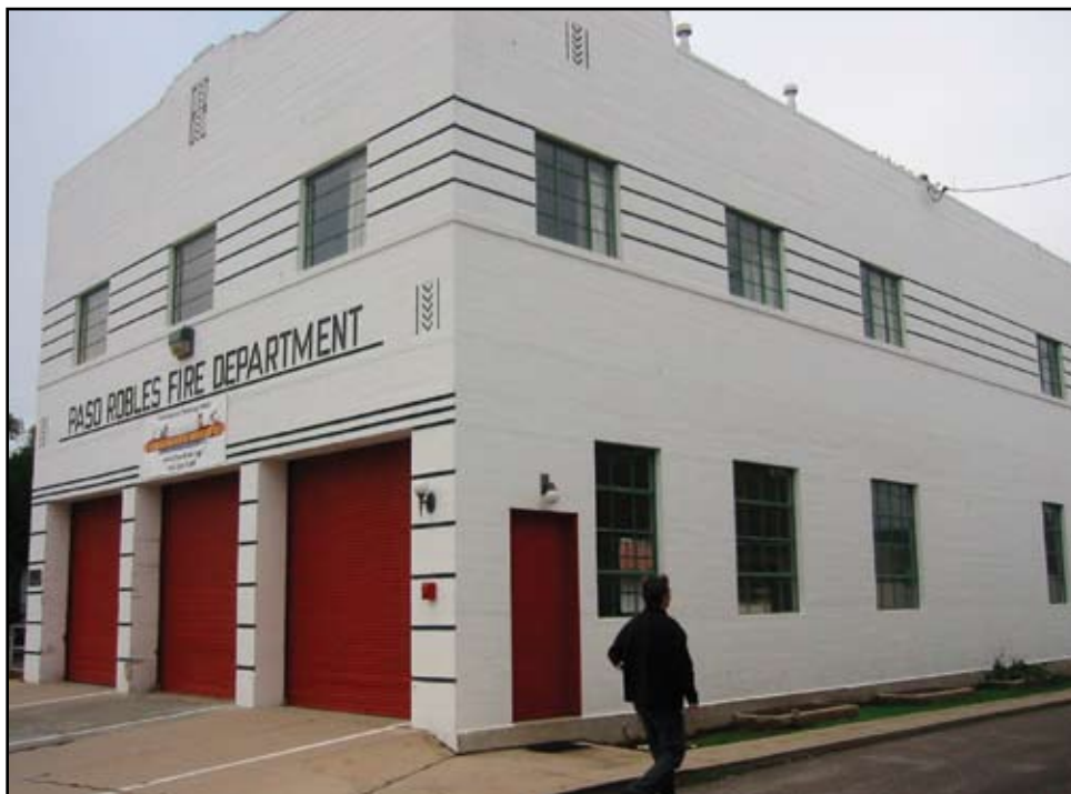
1950s Firehouse located in Paso Robles that also withstood the 2003 earthquake. The second level of analysis, the LDP, is suitable to demonstrate the systems adequacy since there is only a single lateral load path at the first level. Courtesy of Chris Poland, 2003.
