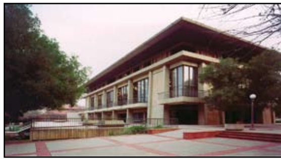
1960s University Library located near Palo Alto, California that was rehabilitated using the third level of analysis, the NSP. By relying on the new cantilever concrete walls located at each corner to arrest the deflection of the building, the existing concrete frame was held to within its limits for safe performance. Courtesy of Chris Poland, 2003.
