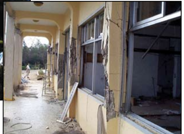
1960s Concrete Weather Station in Taiwan successfully resisted over 125 percent ground shaking without collapse because of the multiple lateral load resisting systems that includes concrete frames and masonry walls. Only the fourth level of analysis, NDP can come close to predicting such performance. Courtesy of Chris Poland, 1999.
