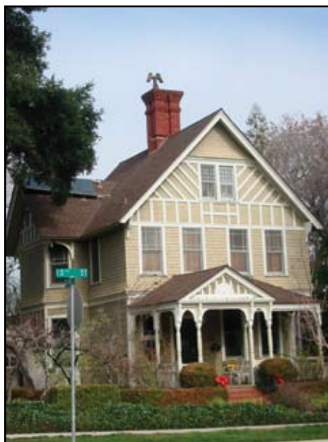
Residence in Paso Robles, California that successfully withstood the 2003 San Simeon Earthquake with limited damage due to its inherent strength and ductility as a wood building and the moderate level of shaking that occurred. The first level of analysis, the LSP, is sufficient. Courtesy of Chris Poland, 2003.
