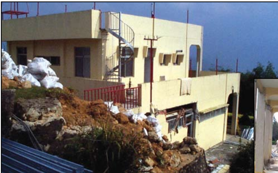
1960s Concrete Weather Station in Taiwan successfully resisted over 125 percent ground shaking without collapse because of the multiple lateral load resisting systems that includes concrete frames and masonry walls. Only the fourth level of analysis, NDP can come close to predicting such performance. Courtesy of Chris Poland, 1999.
