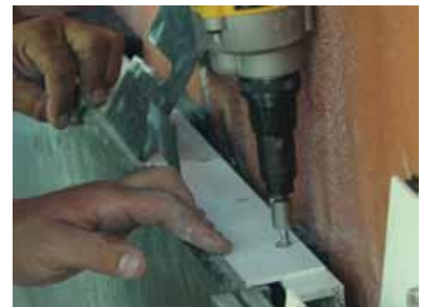
Self-drilling, self-tapping screws install quickly using hand-tools. Courtesy of CDC Curtainwall Design Consulting, Inc.
