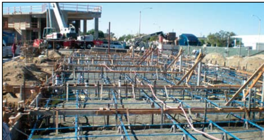
Figure 3: Uniform Thickness Mat Foundation.
