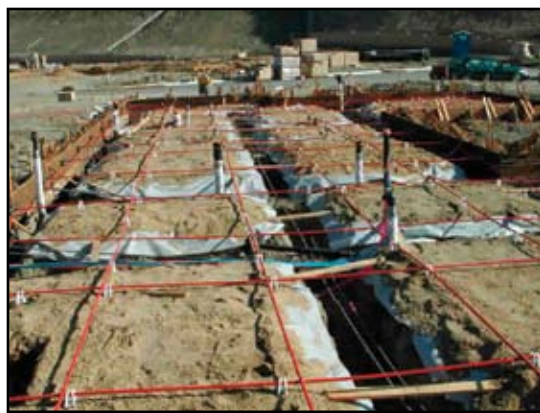
Figure 2: Post-Tensioned Ribbed Foundation.
