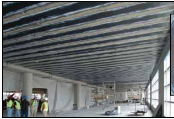
Figure 3: Large Retail Space.
