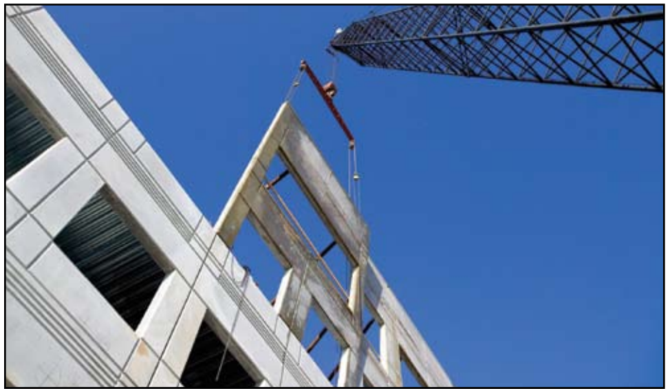
Second tier tilt-up panel lifted into place.
