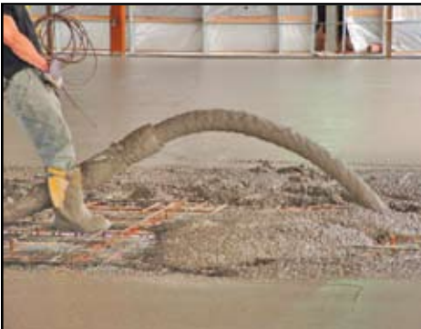
Figure 5: Lightweight concrete being placed on metal decking.
