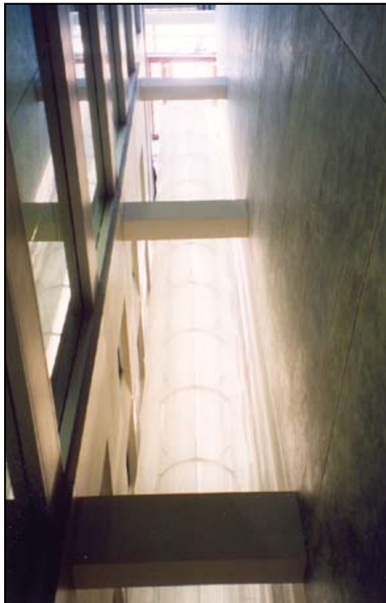
Figure 2: Solar Light Pipe, Washington, DC.
