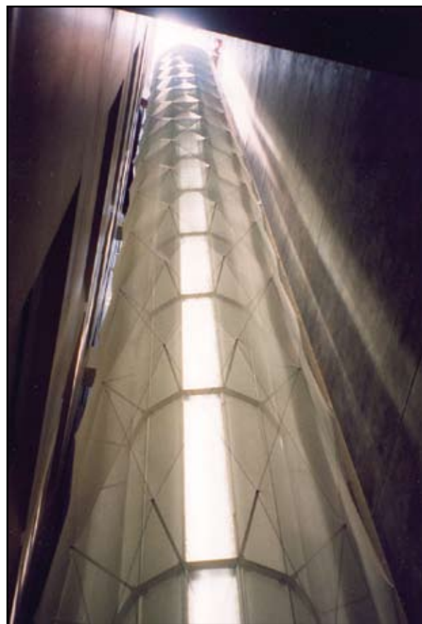
Figure 1: Solar Light Pipe, Washington, DC.
