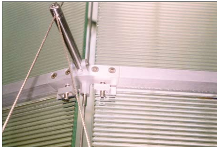
Figure 5: Solar Light Pipe - Typical Glass Connection Detail.
