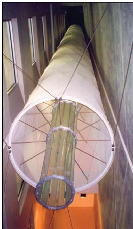
Figure 4: Solar Light Pipe - Bottom Support Ring.
