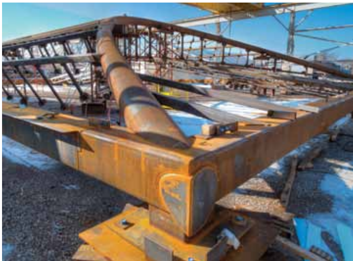
Figure 9. Roof pre-assembly at fabricator's yard.
