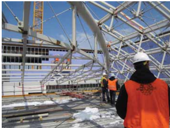
Figure 10. Temporary work platform during roof erection.
