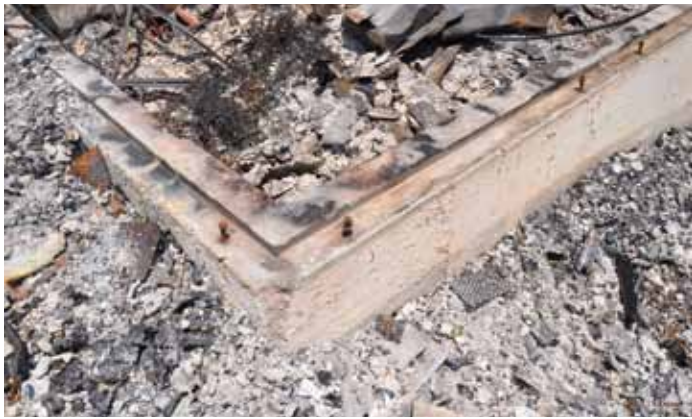
Figures 2 and 3. Views showing how heat-damaged concrete exhibits low strength and crumbles easily when struck four to six times with a hammer. The rebar is exposed, and the fractures are through the paste, not the aggregate. Without conducting any further testing, this foundation is considered not suitable to be re-used in reconstruction of the structure.
