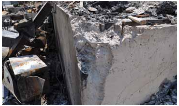
Figures 2 and 3. Views showing how heat-damaged concrete exhibits low strength and crumbles easily when struck four to six times with a hammer. The rebar is exposed, and the fractures are through the paste, not the aggregate. Without conducting any further testing, this foundation is considered not suitable to be re-used in reconstruction of the structure.
