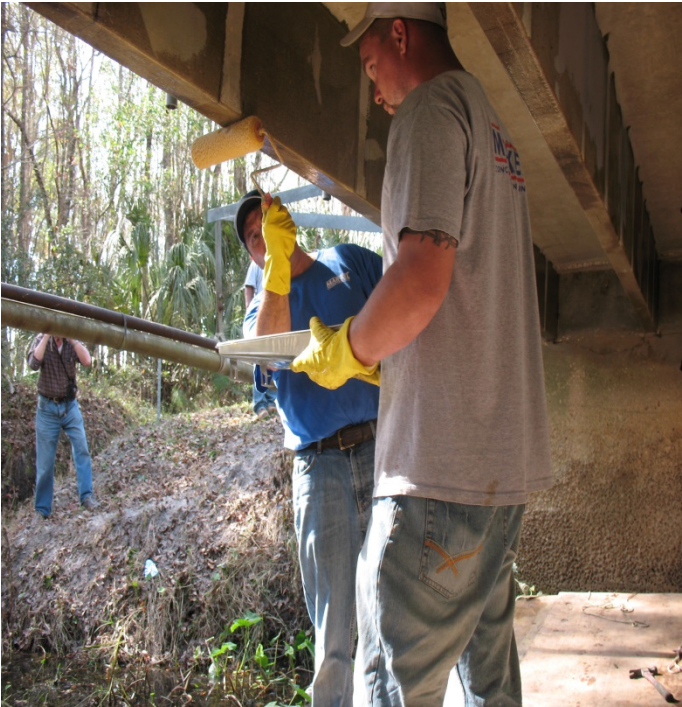
3 – Apply a basecoat of the saturating component
