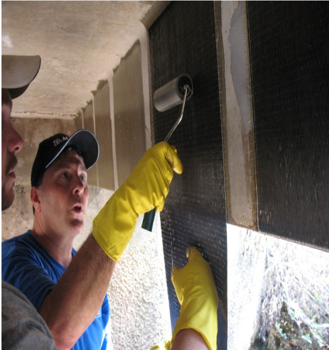
5 – Roll FRP fabric to remove wrinkles & achieve a tight installation
