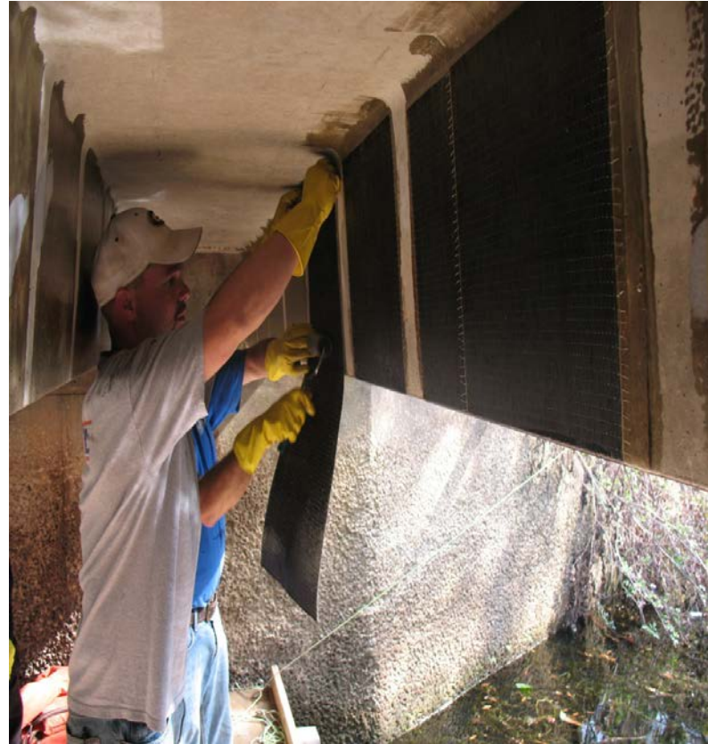
Black Creek Bridge Danbury, CT
