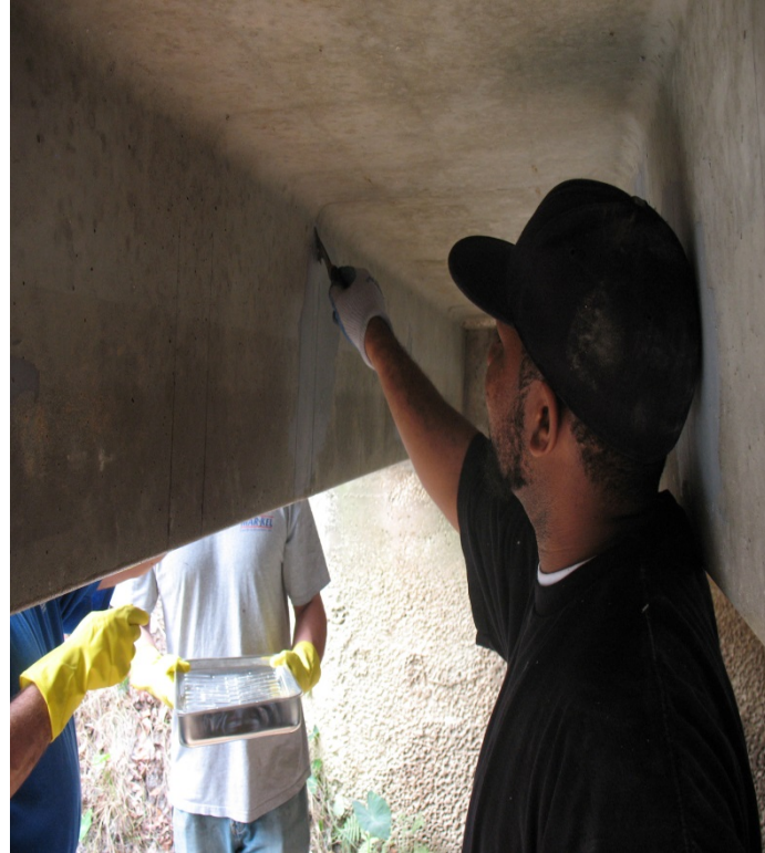
2 - Apply the putty component
