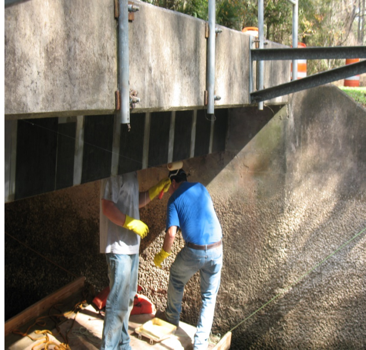
6 – Apply a topcoat of the saturating epoxy component
