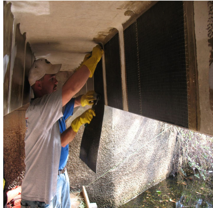
4 - Place the FRP fabric into the still wet basecoat of saturant
