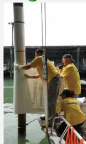
PileMedic™ is the only FRP jacket for repair of deteriorated columns and piles that offers 360 degrees of high confining pressure! It eliminates the need for divers in repair of submerged piles.
