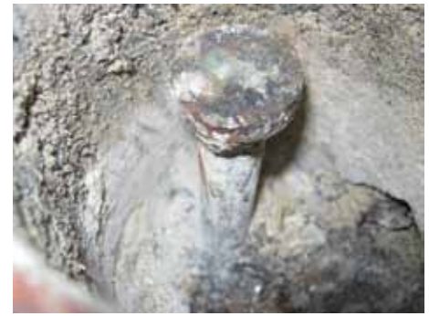
Deteriorated Headed Stud.
