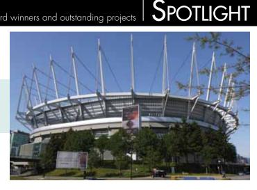
between the radial cables. Pressure in the cushions is automatically modulated in response to roof load. The roof is opened by evacuating the cushions and contracting the membrane into the center gondola of the roof above the new center-hung video scoreboard.
