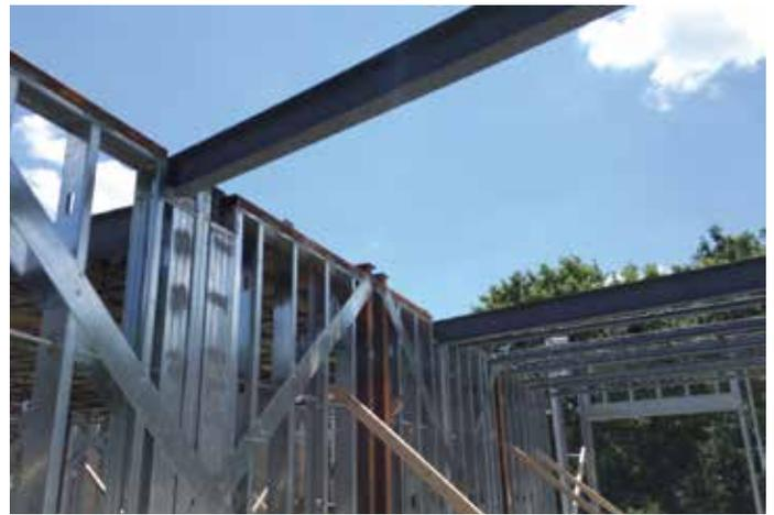
Figure 5. Typical framing with beam pockets.
