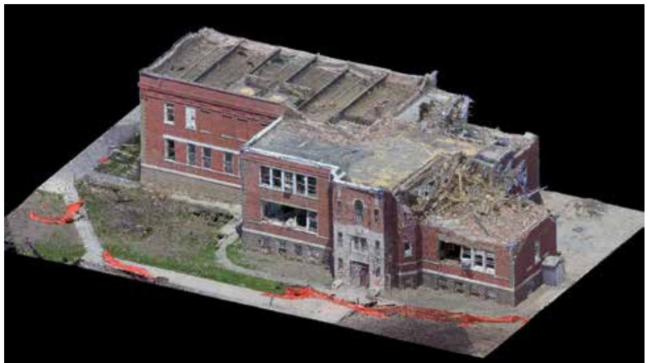
Figure 2. LiDAR scan of damaged school following a tornado. Courtesy of Richard Wood from the University of Nebraska-Lincoln.
