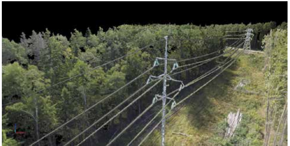
Figure 1. Aerial scan of transmission line using photogrammetry.
