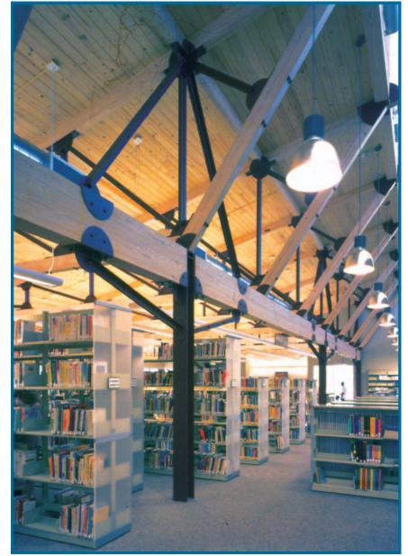
"Glulam trusses and beams were used to add warmth to the exposed structure in combination with steel columns. The use of wood and steel allowed the structure to be fairly open and light, without appearing flimsy or heavy," according to Tom Fennell of Fennel Purifoy Architects in Little Rock.
