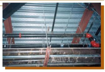
framing is not part of the structural contract and must be included in the MEP contract and specified by the MEP engineer. Alternatively, the MEP engineer can write a performance specification requiring the contractor to hire a structural engineer to design these supports.
