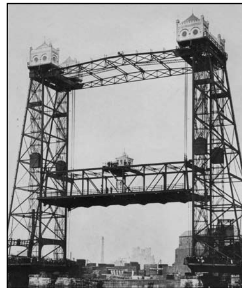
Halstead Street Vertical Lift Bridge, Chicago, IL, 1894, Photo Courtesy of Hardesty & Hanover
