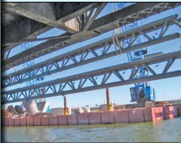
Figure 6: Two cranes on barges lift spliced truss segment into place on pier
