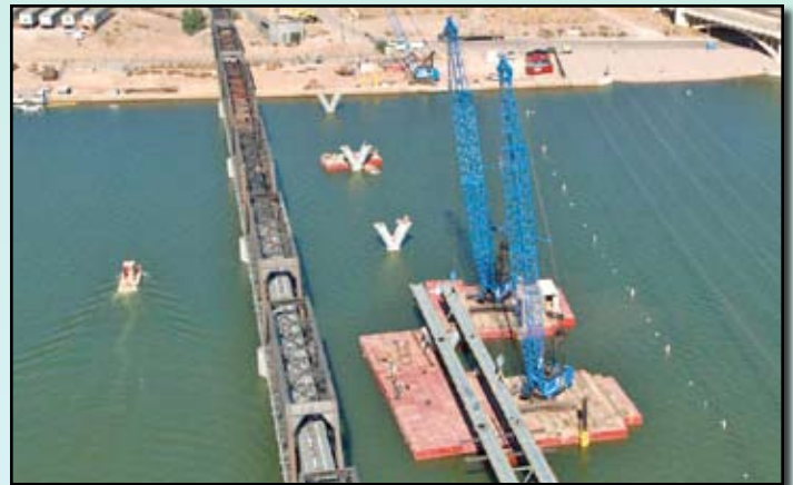
Figure 8: Aerial view looking north as cranes on barges proceed with bridge construction
