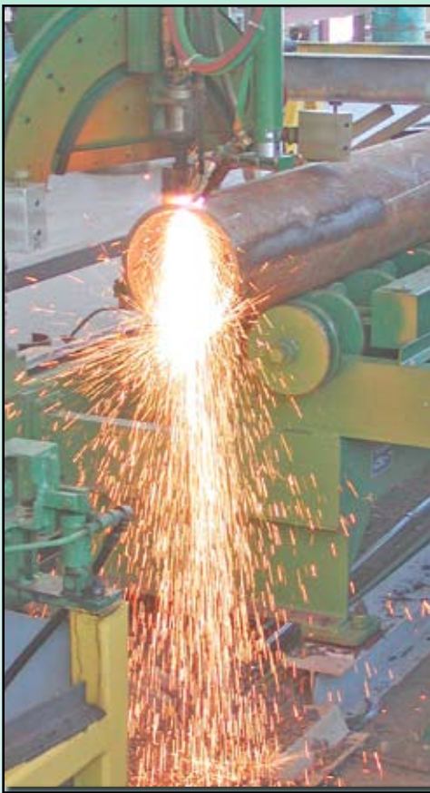
Figure 5: Computer-controlled system cuts the diagonal pipe "fish mouths"
