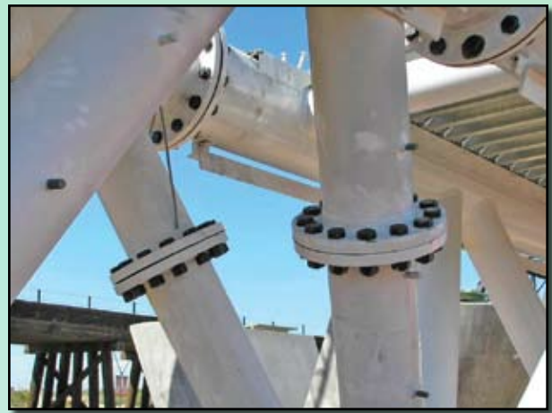
Figure 7: Each splice of two truss segments required 94 bolts
