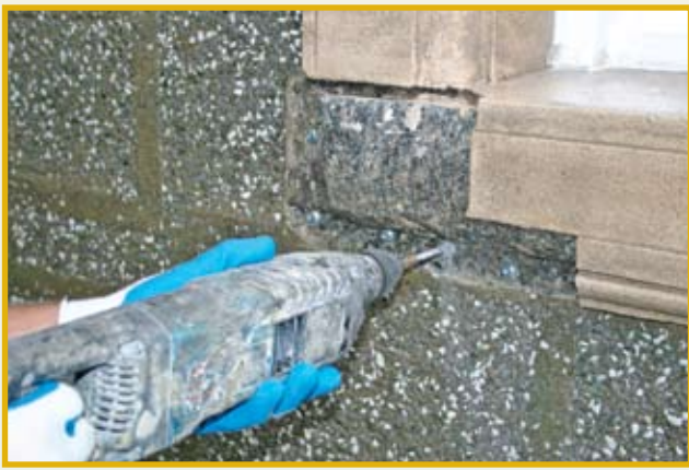
Figure 4: Deteriorated and spalling areas were removed and replaced.
