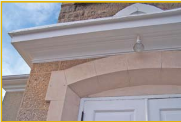
Figure 8: New wood was installed in rotted areas, and the wood in all of the locations was coated with an industrial-grade exterior paint.
