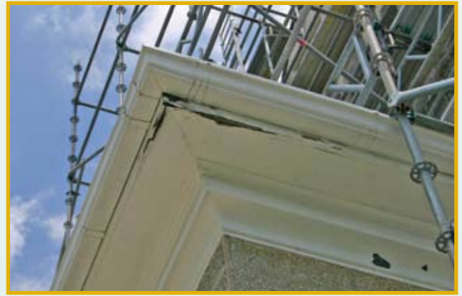
Figure 2: Repairs were also needed for certain portions of the woodwork.
