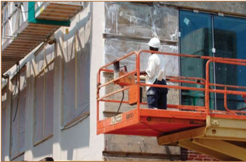
Figure 6: Contractor placing the SACI to the façade via a pump sprayer.
