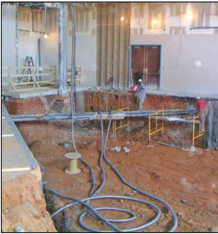
The excavation of the orchestra pit.
