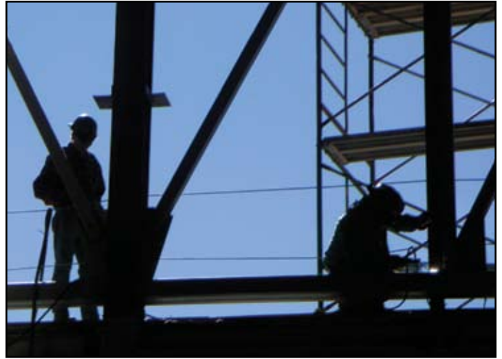
Close-up of the members of the new truss.
