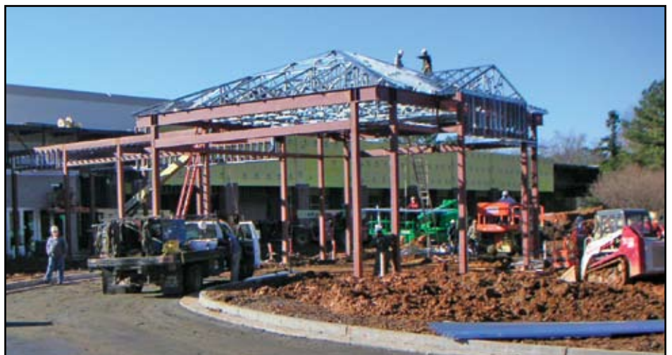
The Port-o-Cochere in progress.
