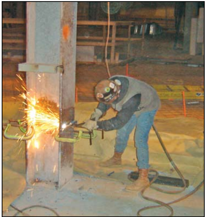
The actual cutting of the load-bearing columns, one carrying over 320,000 pounds.
